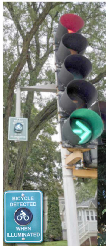
(left) "BICYCLE DETECTED WHEN ILLUMINATED" light and (below) the pavement marker for the sensor registering a biker at the intersection.
