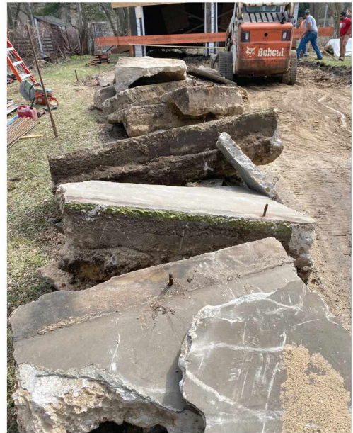
Rubble from the deconstructed garage floor
