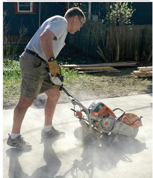
Dennis grinding stress lines into new driveway
