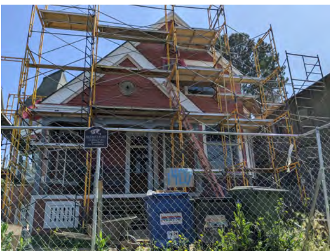
The Winston House, a work in progress
